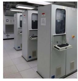
The MicroNet™ Plus control system provides a flexible and expandable platform to control any gas turbine and its associated processes such as system sequencing, auxiliary system control, surge control, monitoring and alarms, station control, and high-speed controls. Digital MicroNet Plus is available in both simplex
